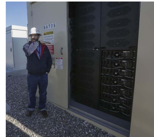
DMP Battery Storage Site
